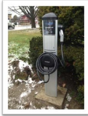
Montpelier, corner of State Street and Governor Aiken Avenue: Example of designated area after installation is complete
